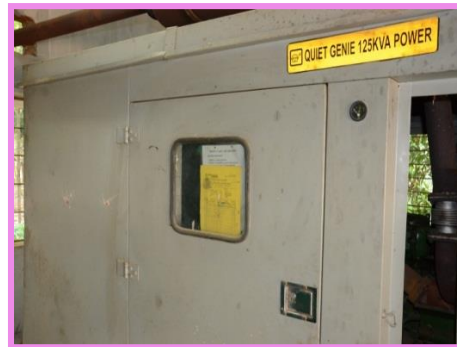
Power Back Up (150 KVA)
